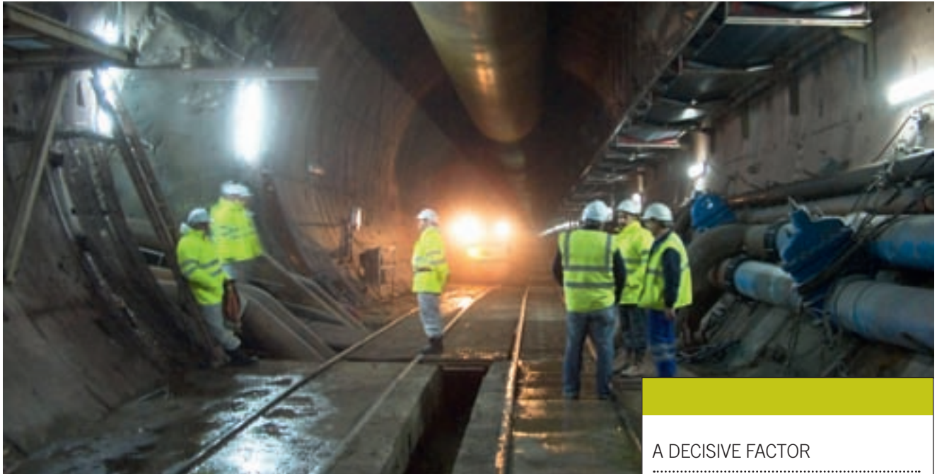
The tunnels have been dug on a downward slope in both the first section, which starts at 1,000 metres above sea-level, and in the second section, whose entry point is halfway up the mountainside.
