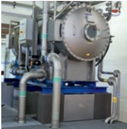
ITT Water & Wastewater's Wedeco ozone generator type PDO 2500 comes into play at Langenau after solid substances have been removed.
